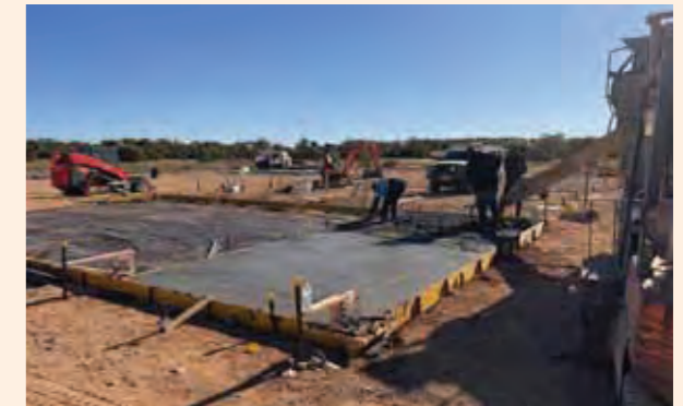
Construction of the Mithaka ranger base
